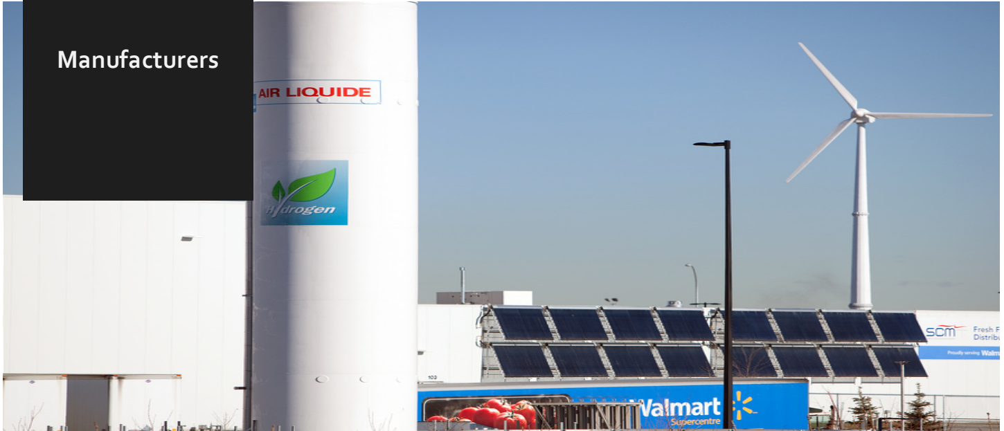
Pictured Above: a distribution center at Walmart featuring on-site wind, solar and hydrogen power. Large retailers are among the market actors that increasingly require sustainability performance disclosure across their supply-chains. Photo credit: Walmart, CC2.0. No endorsement implied.
